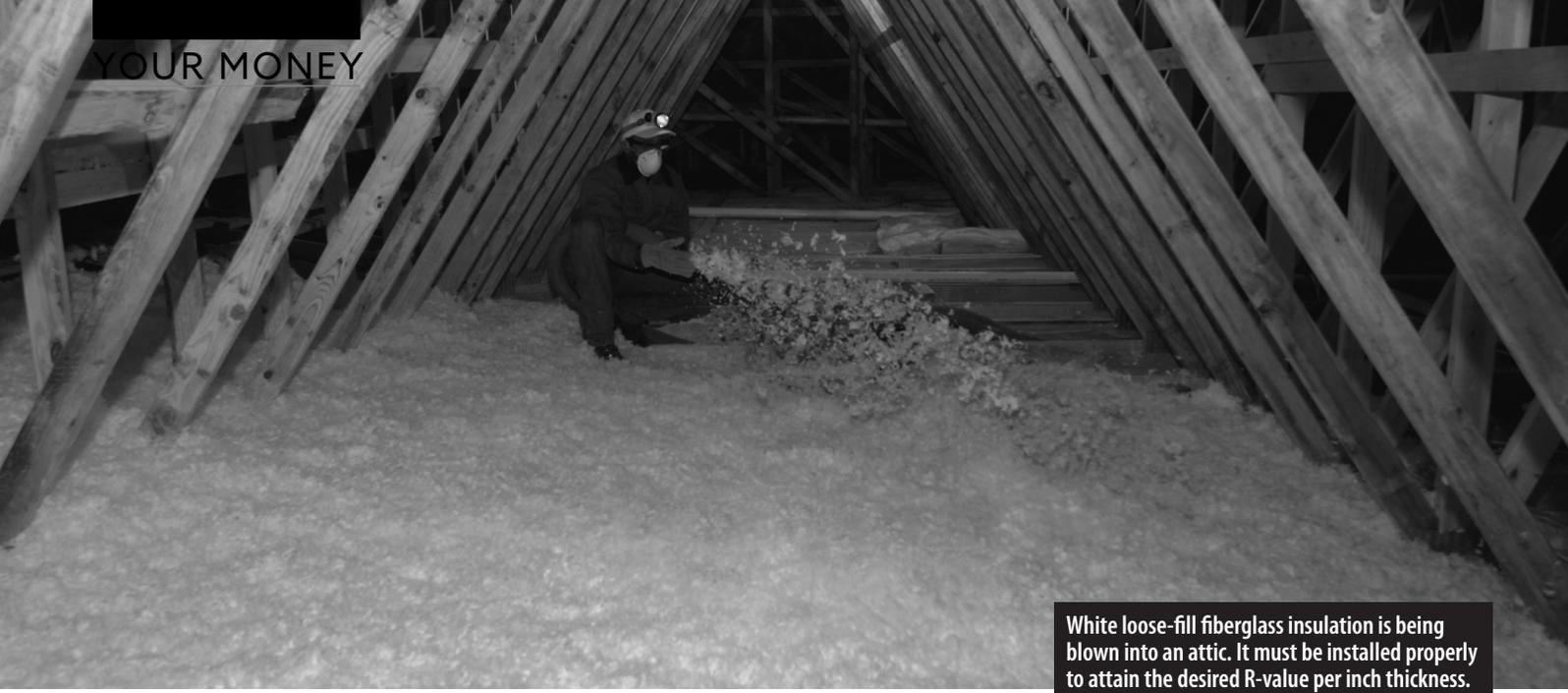
White loose-fill fiberglass insulation is being blown into an attic. It must be installed properly to attain the desired R-value per inch thickness.
